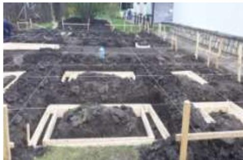
Fig. 7. Belt formwork (*original*)
