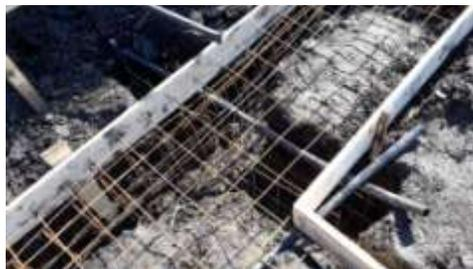
Fig. 8 Welded mesh detail (*original*)
